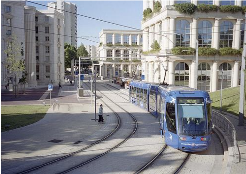
Montpellier Tramway showing the extensive work undertaken to the public realm
